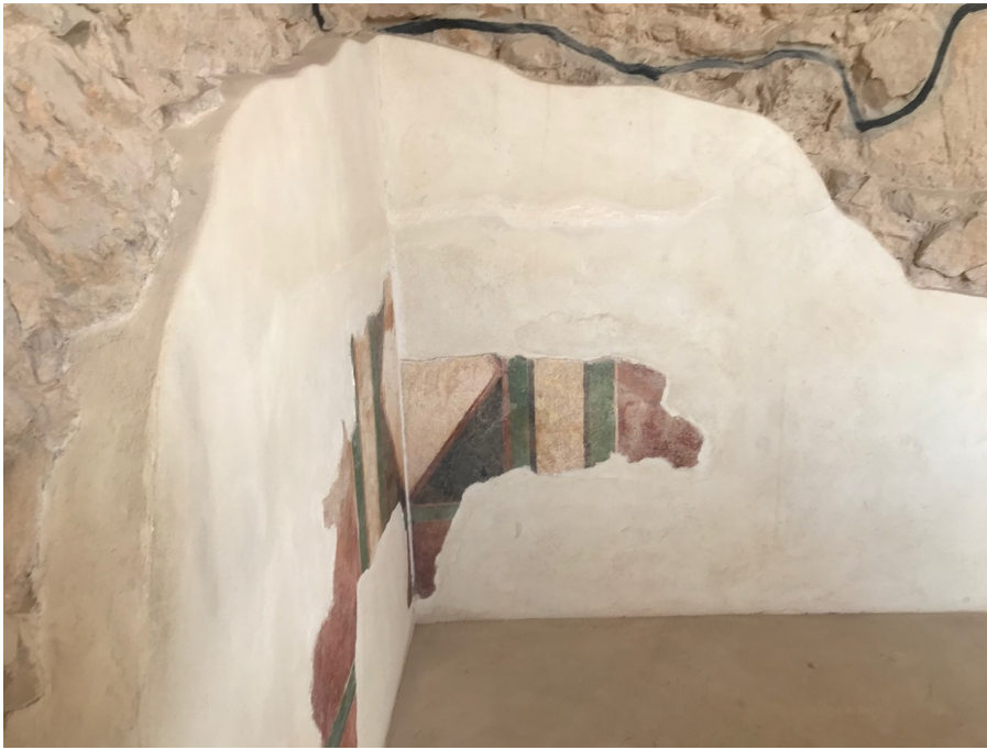
Plaster and Painted Walls at Masada ( photo by Wes Husted )
