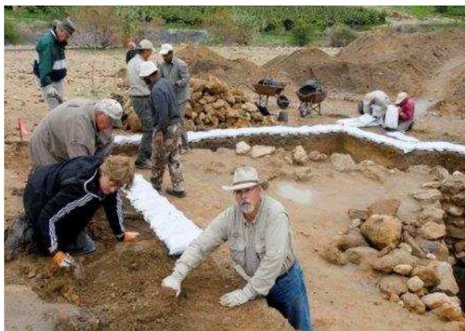
LEVELING UP FOR SANDBAGS
